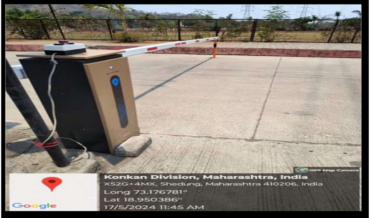
Road Safety Barrier
