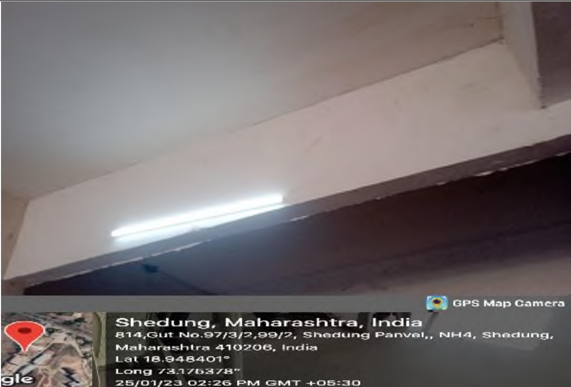
Installation of LED Tube lights throughout the Campus Saving 50% Energy
